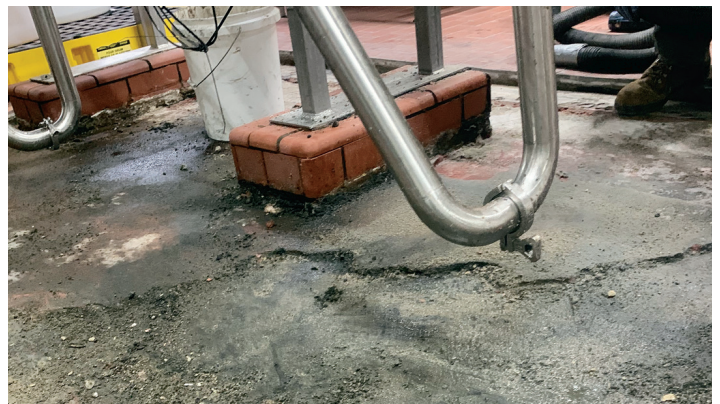
Concrete substrate damage and filth due to missing grout.
