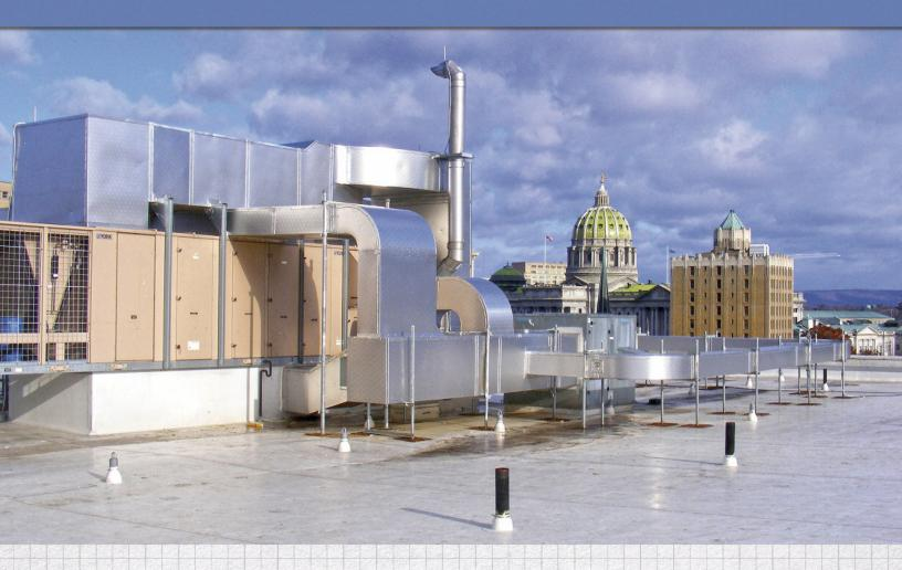
Replacement of failed HVAC ductwork improves energy efficiency and reduces summer cooling hours
