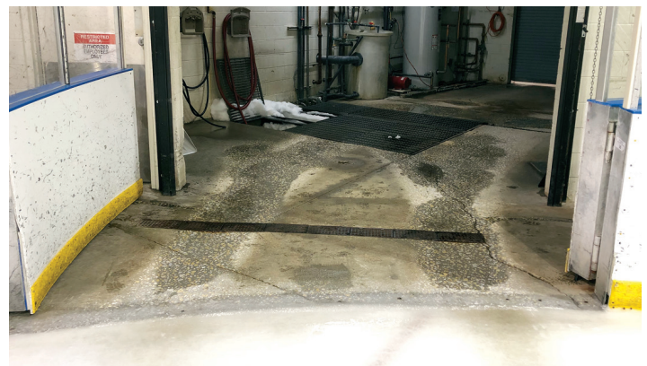
Concrete floor damage from traffic and freeze/thaw effects.
