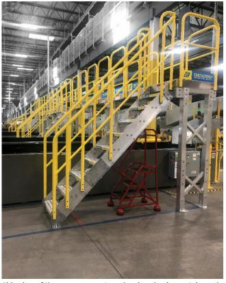
Side view of the crossover system showing aluminum stairs and support structure.
